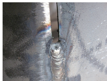
(a) 封底焊出现气孔和裂纹
