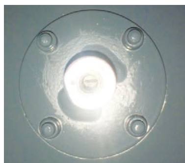
(a) 接地螺钉环槽铆钉铆接
