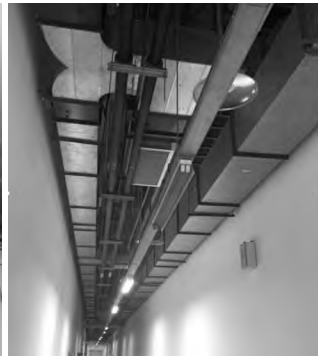
图5 变电所左侧走廊桥架现状 Fig. 5 Corridor trunking on the left side of substation present situation
