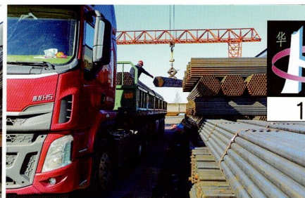
钢管外运 Transportation of steel bar for prestressed concrete
