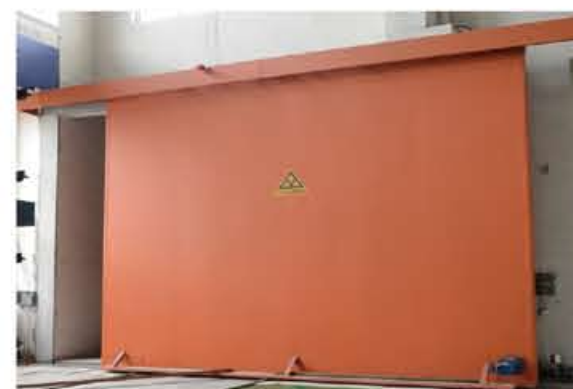
射线探伤室 X-rays Flaw Detection Room
