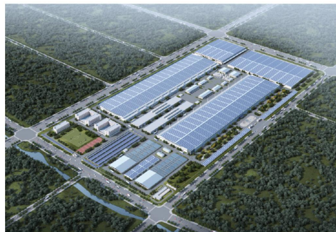
► Chahe New Energy Industrial Park, Chuzhou, Anhui
