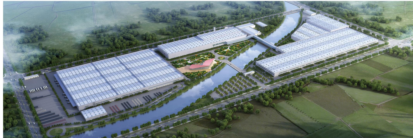
► Anqing Smart Industrial Park, Anhui
