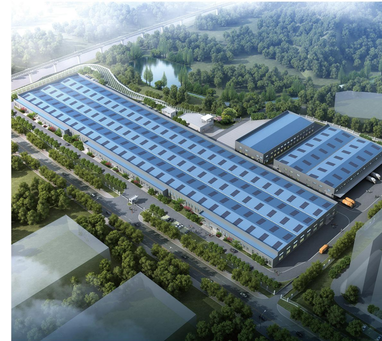
► Lens Technology Laser Smart Manufacturing Plant
