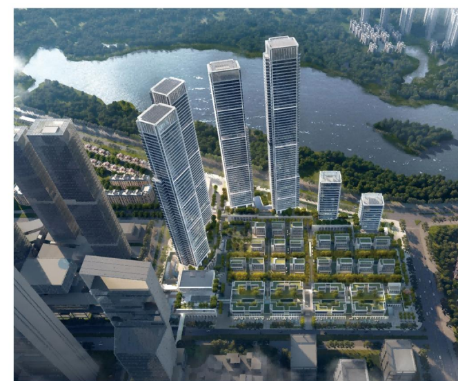
► Shenzhen Bay Coastal Business Center
