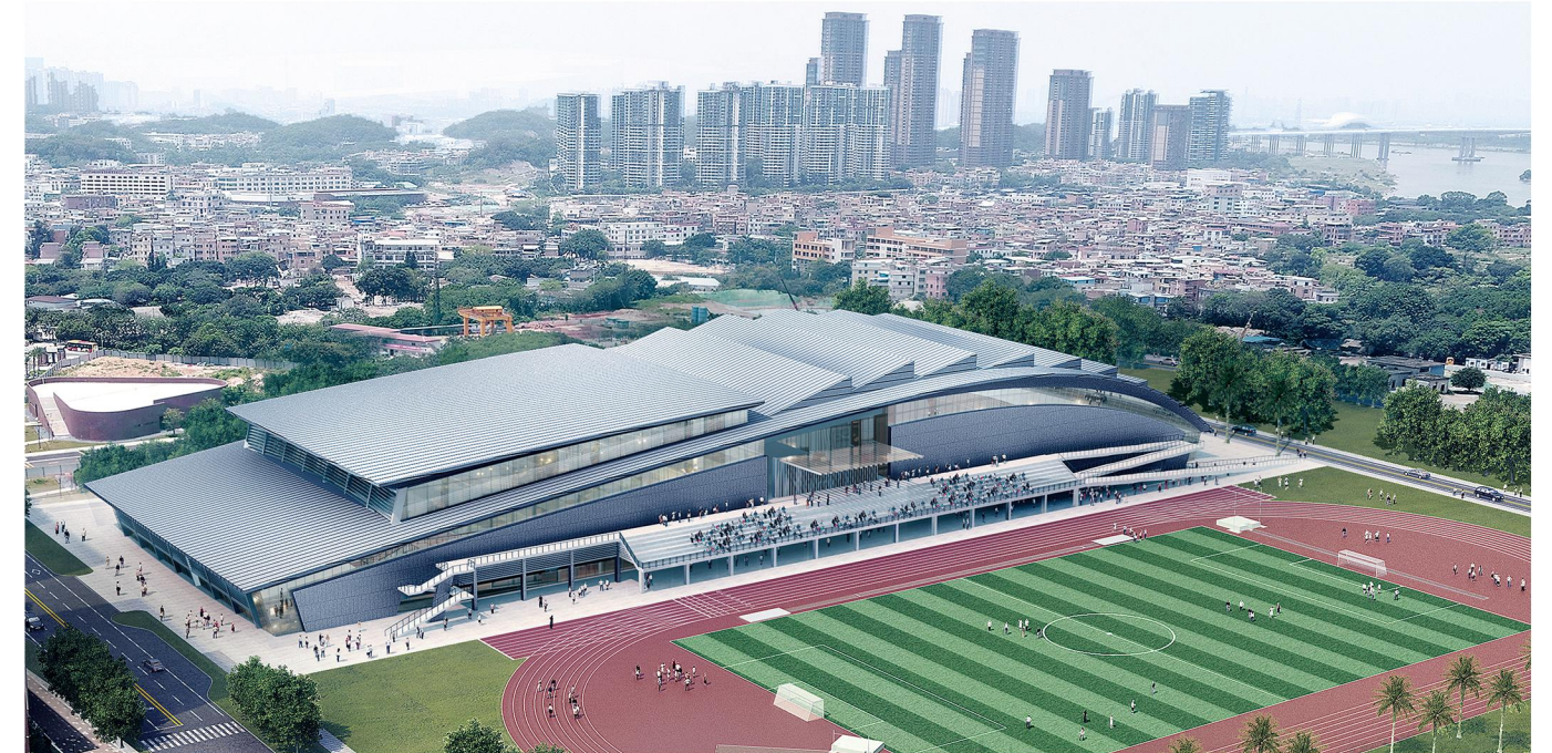
► Guangzhou International Campus, South China University of Technology Winner of the 2022 Golden Waterproof Award (Gold Prize) - Science & Technology Award for Engineering Excellence in Building Waterproofing Industry
