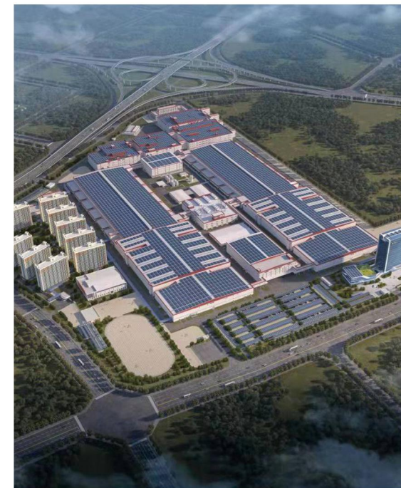
► CATL Xiamen New Energy Battery Industrial Base
