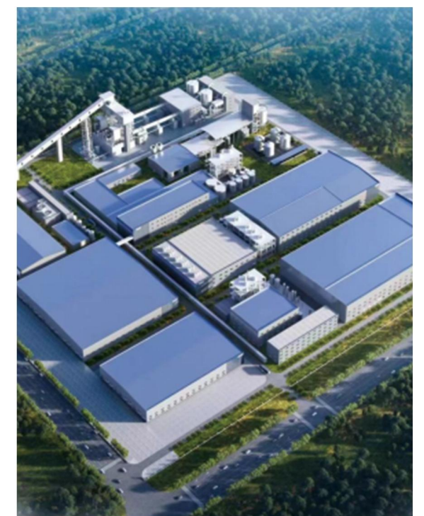
► Huayou 50,000-ton Battery-grade Lithium Salt Plant, Guangxi
