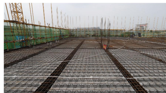
钢筋桁架免拆楼承板修补
